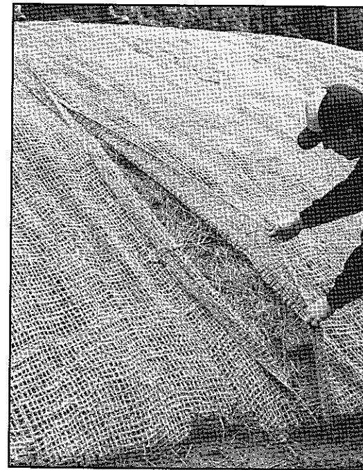
Slope seeding with long straw mulch and jute matting
