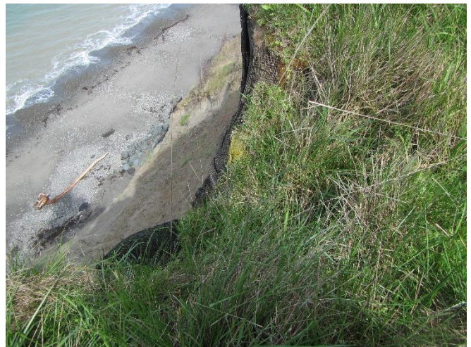
Photo 6. Looking towards beach from 192 Cypress Cir.
