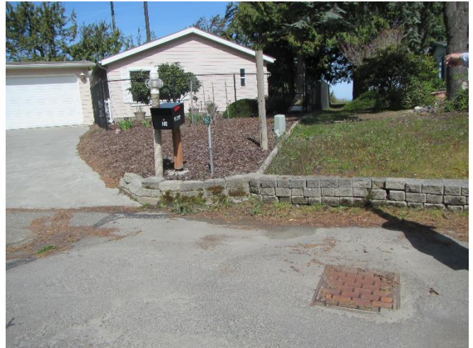
Photo 10. Drainage culvert at 162 Cypress Cir, looking towards bluff.
